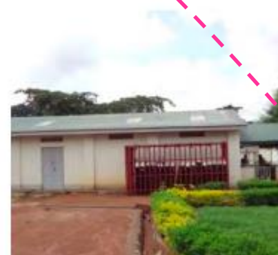
8. Stock yard for oxygen gas bombs with proper guarding.
